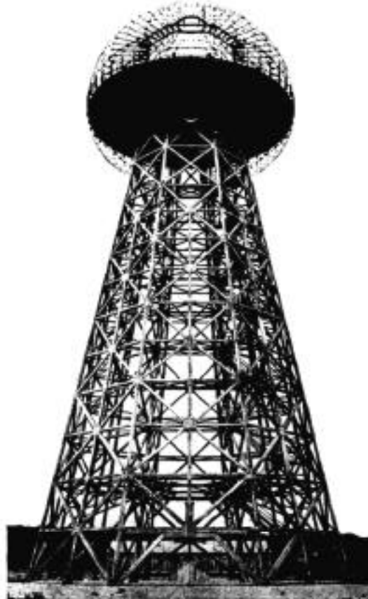
Tesla's 187-foot Wardenclyffe Tower in 1903; it stood unfinished for the next 14 years. The two-storey power plant is in the background.
